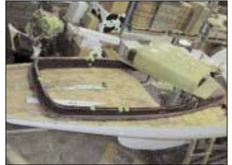
The deck repair on Windfall, NZL12
